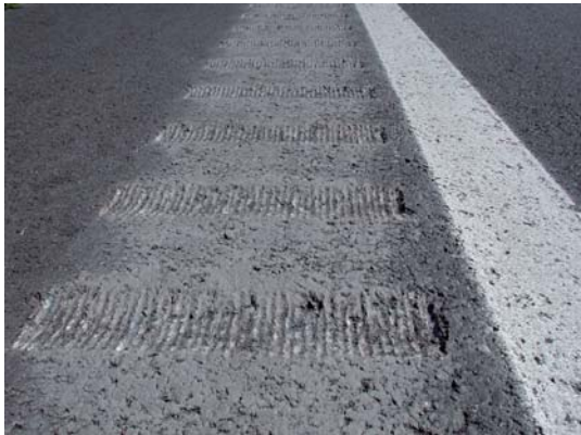
Photo 2-10: Rumble strip at the shoulder
