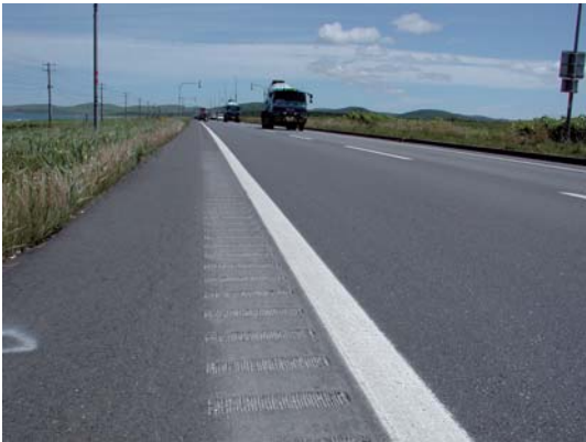
Photo 2-9: Rumble strip at the shoulder
