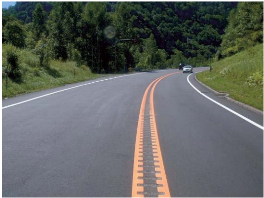
Photo 2-5: Rumble strip at a no-passing double-yellow centerline section
