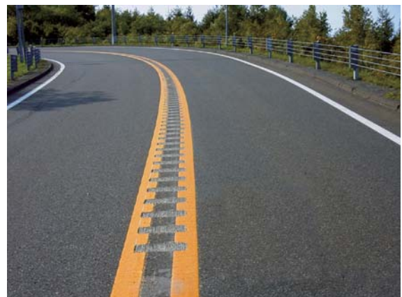
Photo 2-2: Rumble strips installed temporarily at a sharp curve
