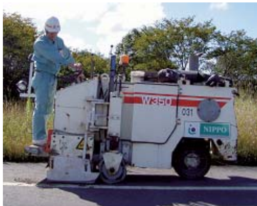
Photo 3-1: Rumble strip installation machine
