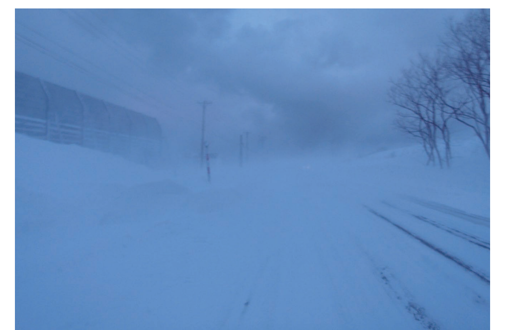
▲防雪柵端部の視程障害 Visibility reduction at the end of a fence
