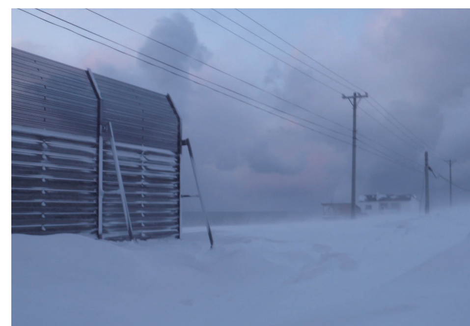
▲防雪柵端部のふきだまり Snowdrift at the end of a fence
