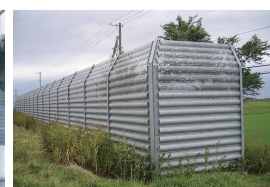
▲防雪柵の端部対策例 Examples of treatments for snow fence end parts
