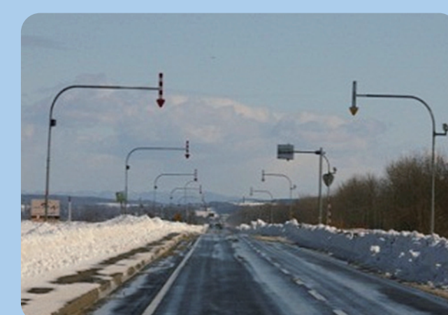
固定式視線誘導柱(矢羽根) Fixed-post delineator (with arrow-shaped pointer)
