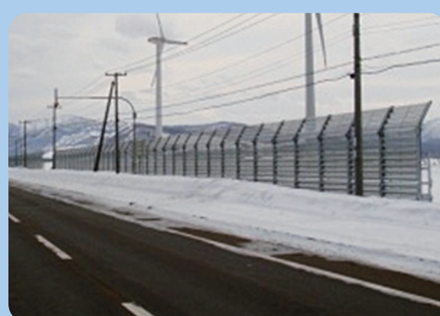
吹き止め柵 Collector upwind snow fence
