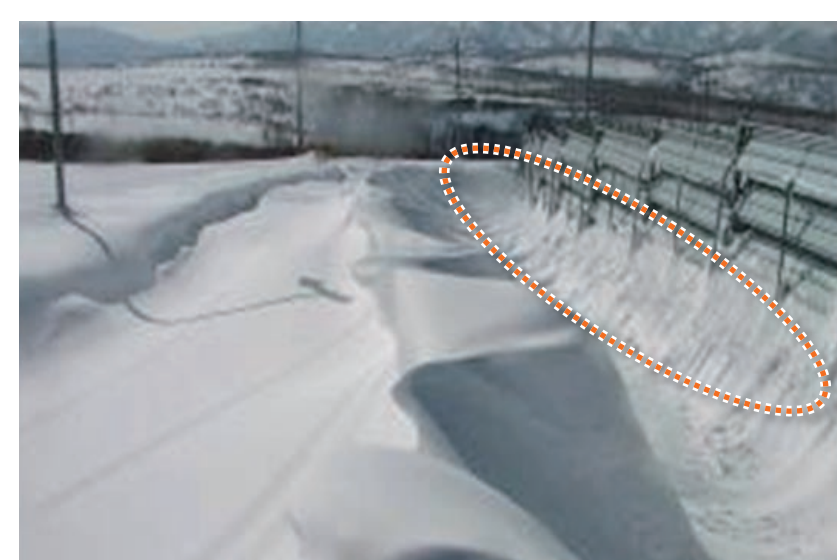
▲下部間隙閉塞時の吹きだまり Snowdrift created when the bottom gap is blocked
