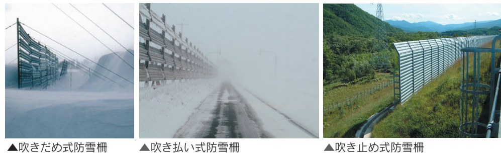
▲吹きだめ式防雪柵
