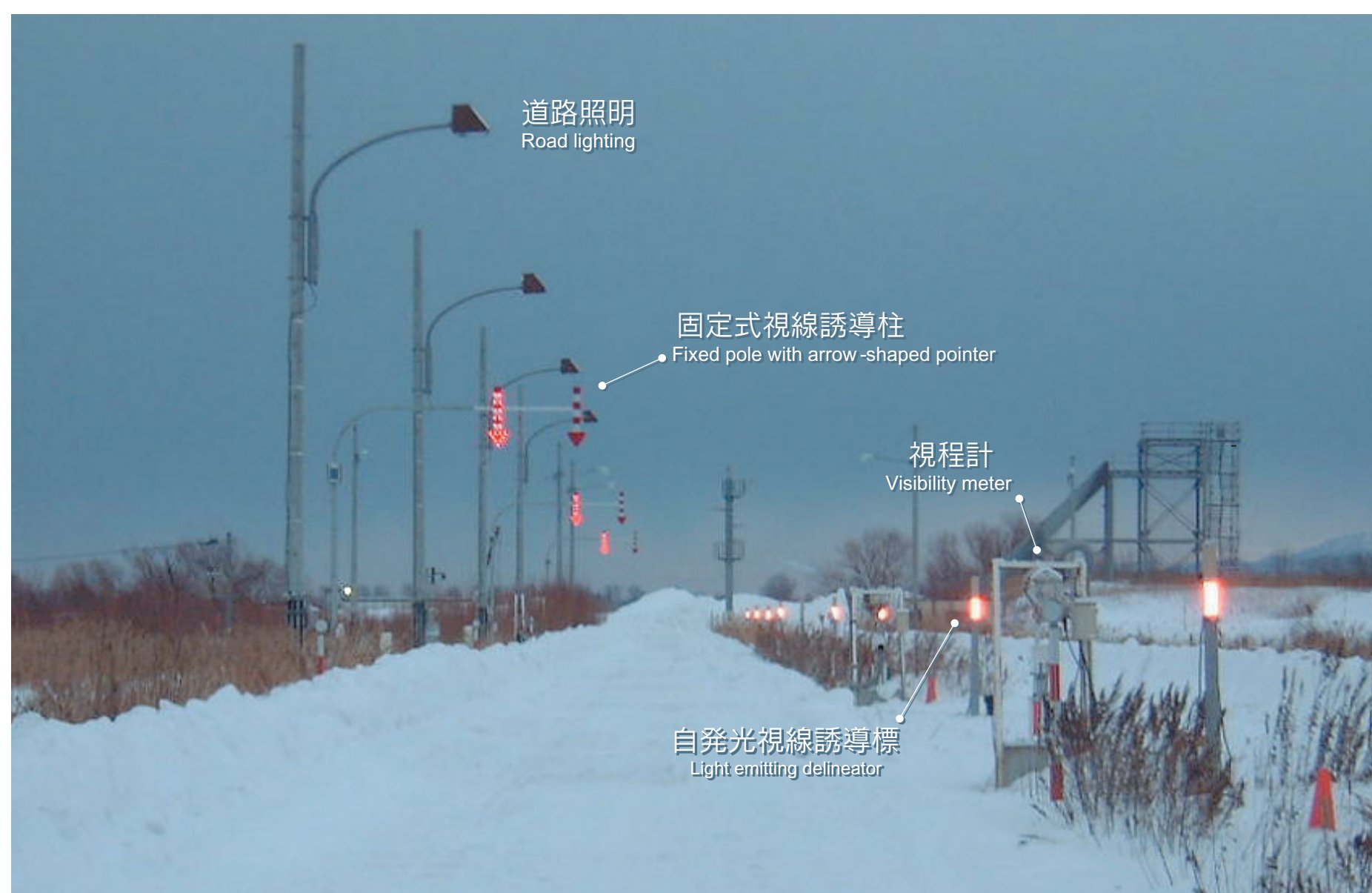
▲試験道路直線部の道路付属施設設置状況 Road facilities installed along the straight section
