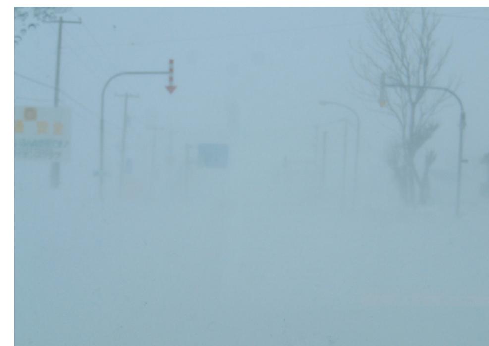
▲固定式視線誘導柱 Delineators with over-hanging arrow
