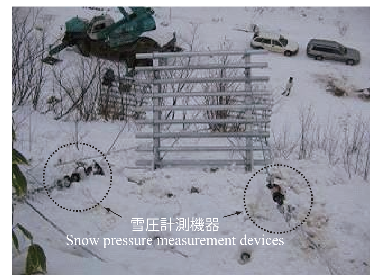
▲雪圧の測定状況 Observation of snow pressure
