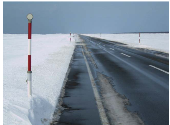
Photo 4-3-2 Retractable Delineator
