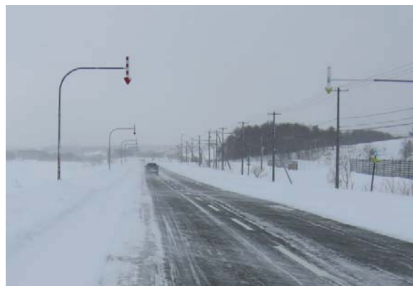
Photo 4-3-5: Fixed-post Delineator with Arrow-shaped Pointer
